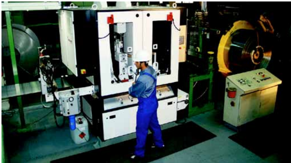
Another close up of machinery installed at Vogel-Bauer Edelstahl.
