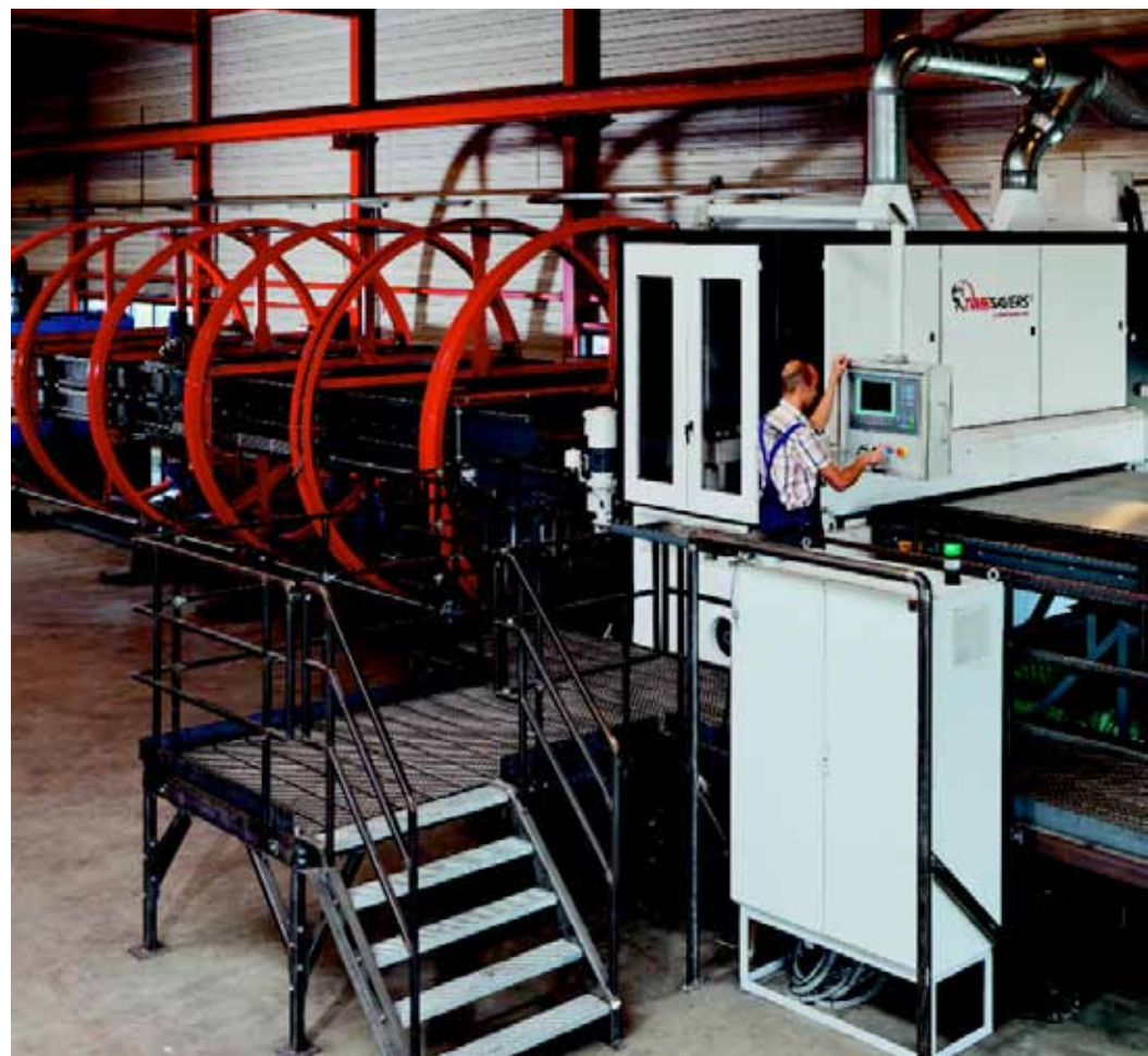
Timesavers machinery installed at Cemilas B.V. in Sint Maartensdijk, The Netherlands.
