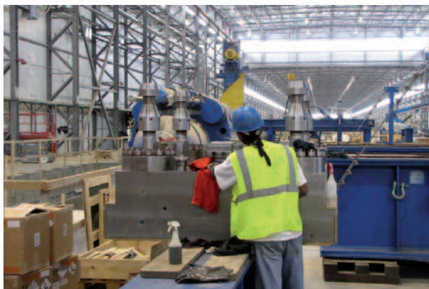
Installing machinery will soon be complete.
