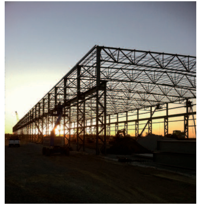
Construction started after groundbreaking in March 2010.
