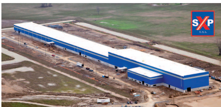
SXP's in-line production will take place in a production hall which is longer than 400m.
