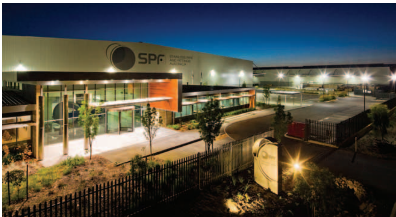
The exterior of SPF's West Australian site including office, warehouse and distribution facilities.
