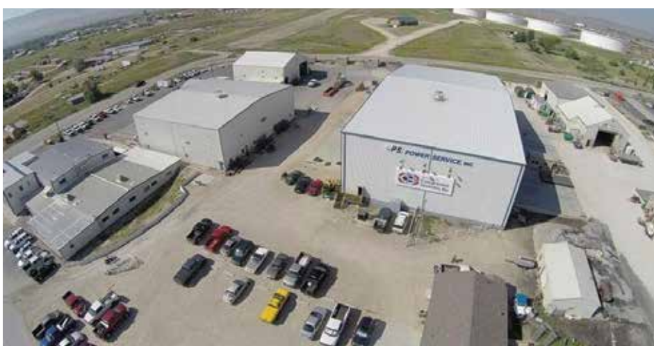
DistributionNOW's recently acquired Power Service location in Casper, Wyoming.
