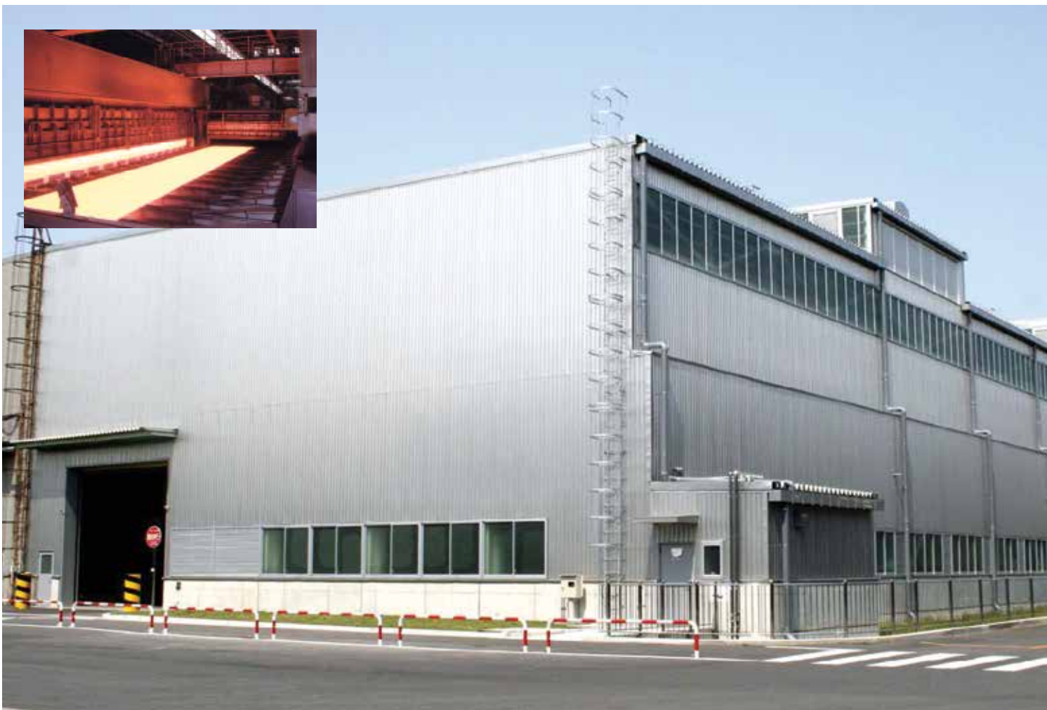
Nippon Yakin's plate mill at Kawasaki, showing as an inlay (top left) its plate heat treatment furnace.
